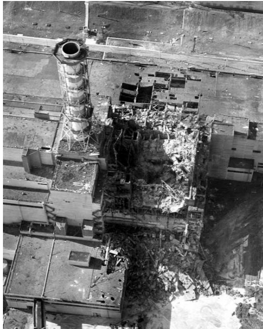
Explosion Aftermath – Helicopter View – 1986
