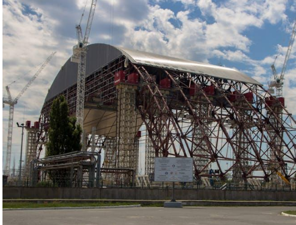
Building the New Safe Confinement
